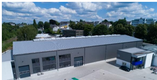
Technical center with milling operation, quality & testing facility, injection molding and lab extruder
